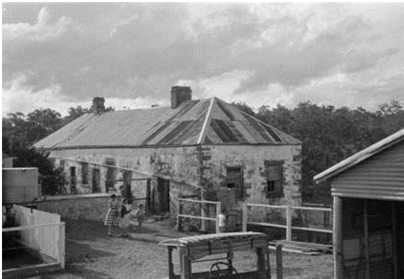
FIGURE 11. THIS BUILDING APPEARS TO BE "VICTORIA INN" BEFORE IT LOST ITS ROOF, CHIMNEYS AND WINDOWS. (NATIONAL ARCHIVES OF AUSTRALIA) 41
