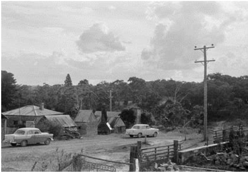
FIGURE 9. NATIONAL ARCHIVES IMAGE 3. THE SAME STRUCTURES IN FIGURE 9 SEEN FROM ACROSS THE ROAD. (NATIONAL ARCHIVES OF AUSTRALIA) 39
